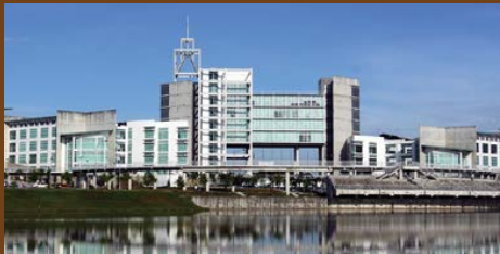
View of UNIMAS Administrative Building
